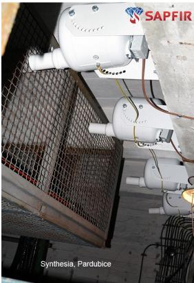
Autonomous dry powder extinguishing SAPFIR is ideal for extinguishing electrical equipment, electronics and almost anywhere but it MUST NOT come into contact with water! Extinguishing is resistant to outside temperature in the range of -60 to + 125  $^{\circ}$  C! It has proved especially successful in extinguishing hydraulic lines, which are the most common source.
