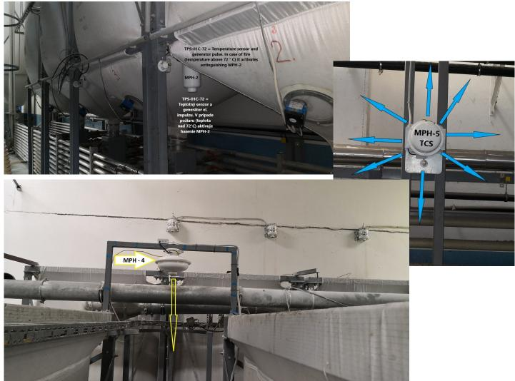
**STOP-FIRE-SAPFIR** autonomous fire extinguishing systems are used for extinguishing all types of electrical equipment. They are designed for extinguishing narrow and long cable ducts, as well as electric transformers and wind power plants up to 40,000 V.
